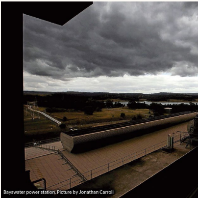
Bayswater power station. Picture by Jonathan Carroll
